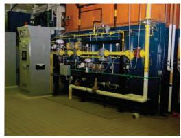
Lipten's scope also included a re-furbished triplex softener system, a new power distribution system, three new burner management & combustion control systems, a plant master system and a dual PLC based plant monitoring system. An entirely new instrumentation control valve and control device package was also included. Lipten provided engineering, project management, start-up, training and commissioning.
