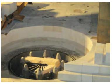
The stoker was removed and replaced with a floor built of plate steel and refractory. This image shows the vertically mounted burner and new floor.
